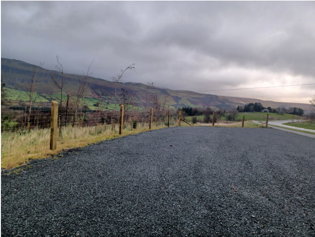
Figure 2: N16 Lugatober – Additional fencing at Collinsford
