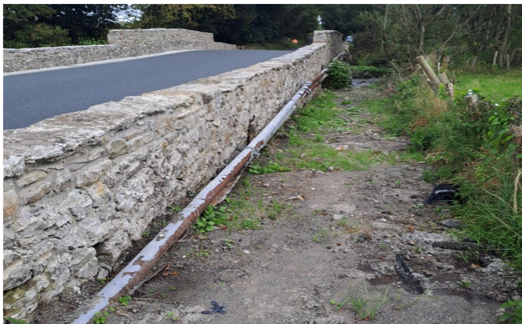
Figure 24: Closkeybeg Bridge Post-Construction Works
