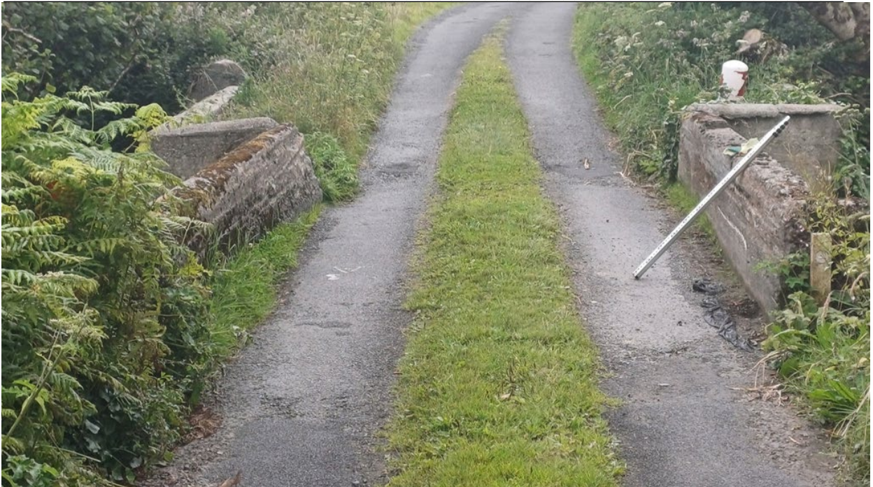
Figure 21: Taylors Bridge Pre-Construction Works
