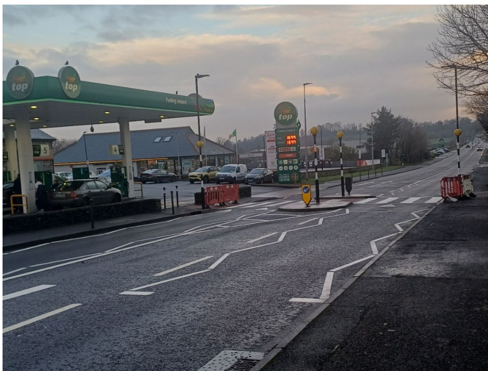
Figure 5: N15 Shannon Eighter (HD15) Pedestrian Crossing RSIS - Completed in 2025
