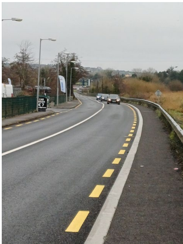
Figure 11: Road resurfacing works on the L3608-0-S0
