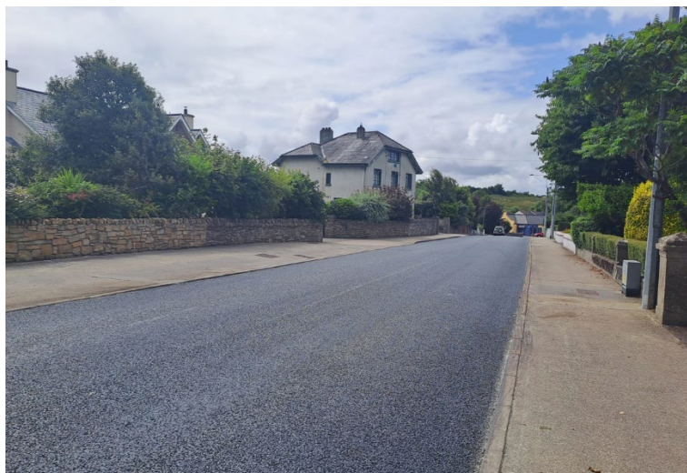
Figure 9: Road Resurfacing Works at Hazelwood Road, Sligo 2025
