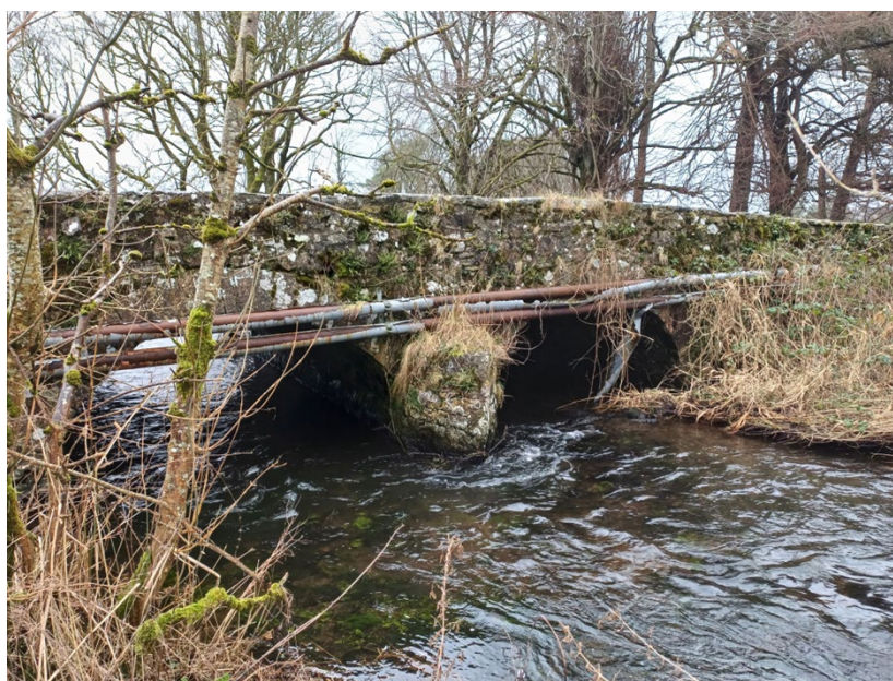
Figure 23: Closkeybeg Bridge Pre-Construction Works
