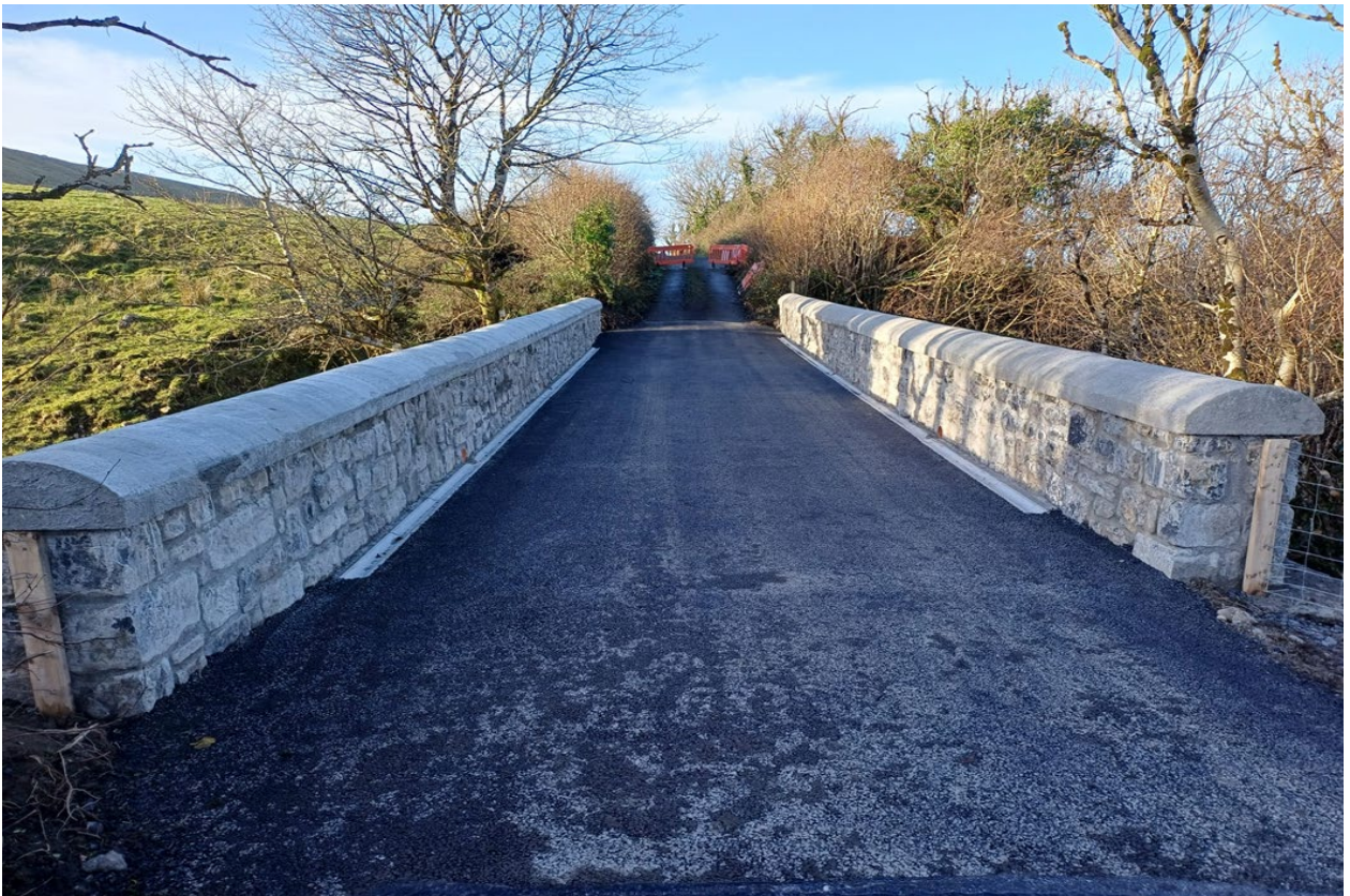
Figure 22: Taylors Bridge: Post-Construction Works.
