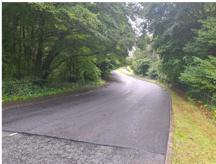
Figure 10: Road Resurfacing works at Cleveragh Drive, Sligo 2025
