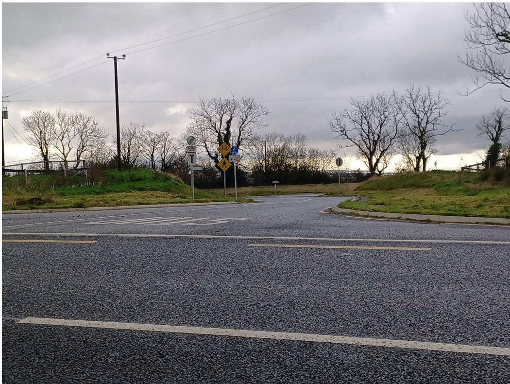
Figure 3: N16 Lugatober – Additional signage at L47311
